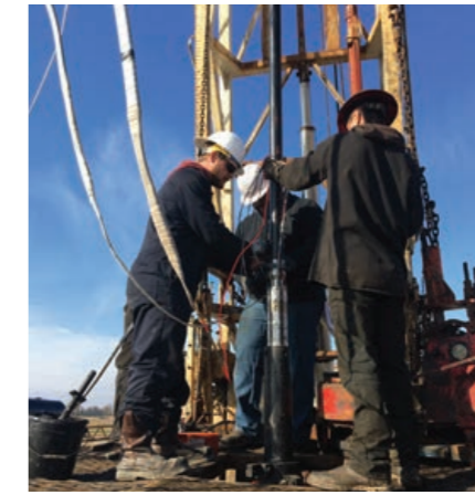
Shroud Installation to Handle the Extended Length of the Tailpipe
