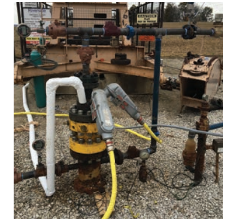
Wellhead after Installation and Instrumentation
