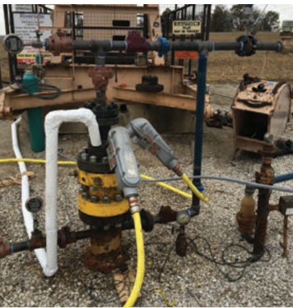
Wellhead after Installation and Instrumentation
