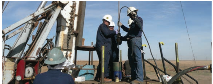
SCS proof-of-concept trials sucker rod deployment
